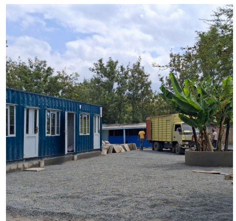
A shipping container transformed into staff quarters and a sick bay now provides safer care and rest at Garden of Eden.
