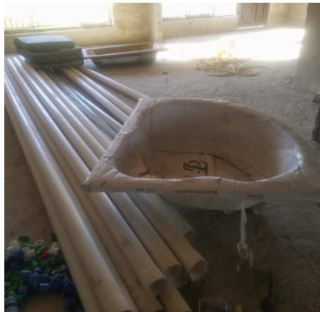
The new Mab's Haven home is nearly ready, with essential systems, furnishings, and safety features now in place.
